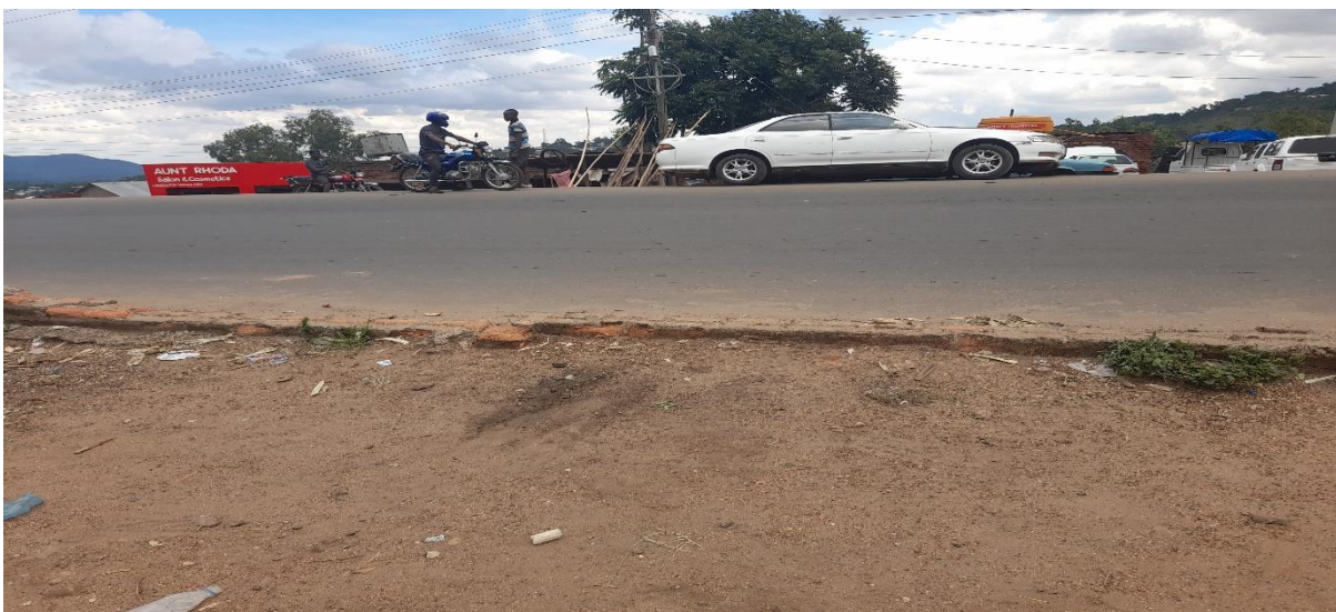
Figure 6: Improved shoulders and drainage system between Kandodo corner shop to Zalewa
