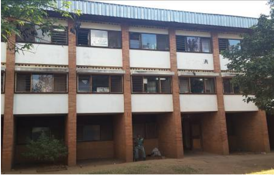
Hostel window fittings also made of timber fittings and exposed to outside environment
