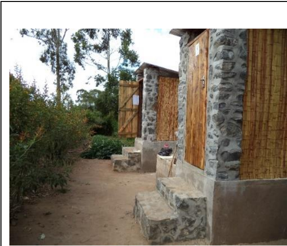
Figure 16: TPS Toilet Structure
