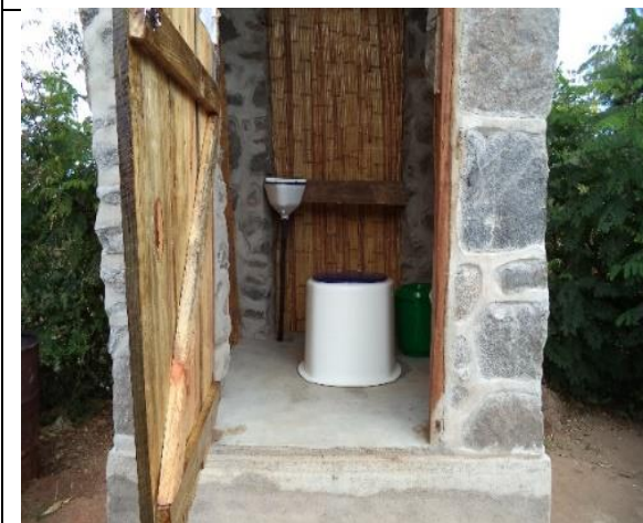
Figure 18: TPS Toilet Inside
