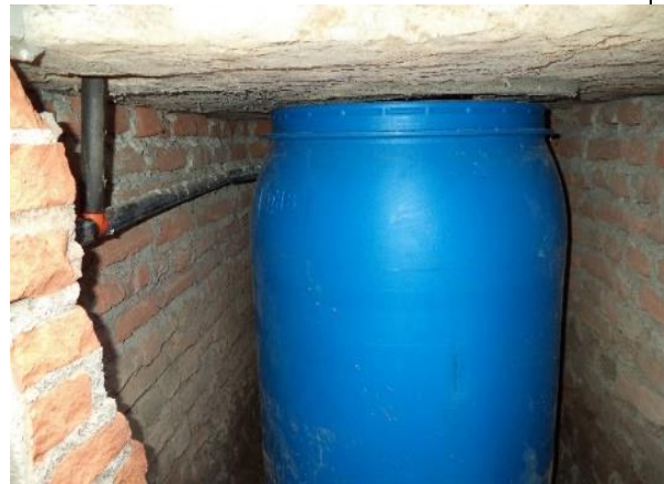
Figure 19: TPS Urine Diverting Pipe Network
