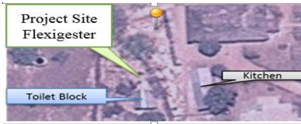
Figure 12: Anaerobic Digester Site; Aerial View
