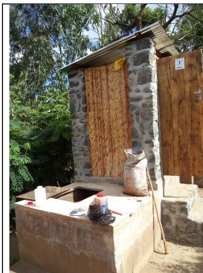
Figure 22: Manhole and Super Structure
