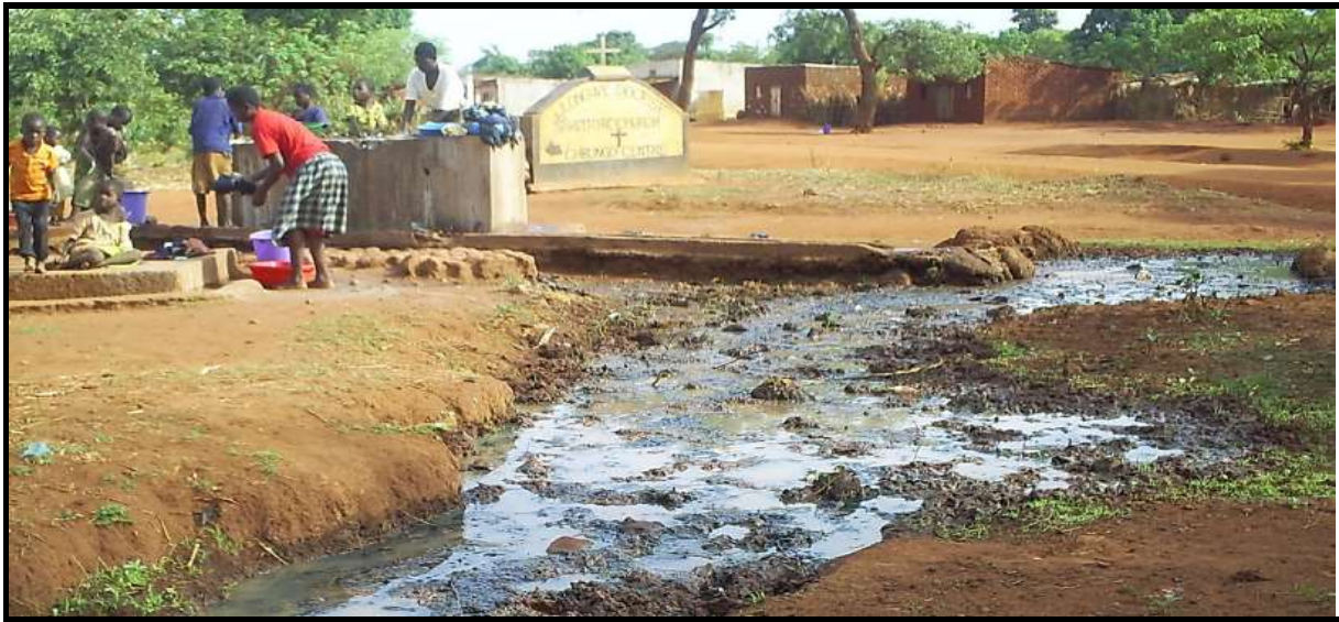
Figure 28: Poor Wastewater Disposal
