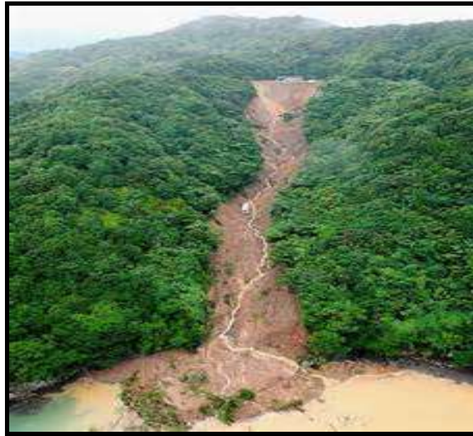
Figure 30: Overflow from Open Conduit Causing Landslides
