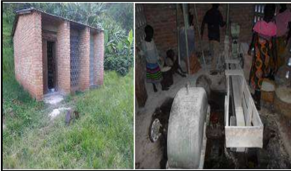
Figure 26: Maize Mill Powered by Water from the Scheme Water Source Reservoir Tank
