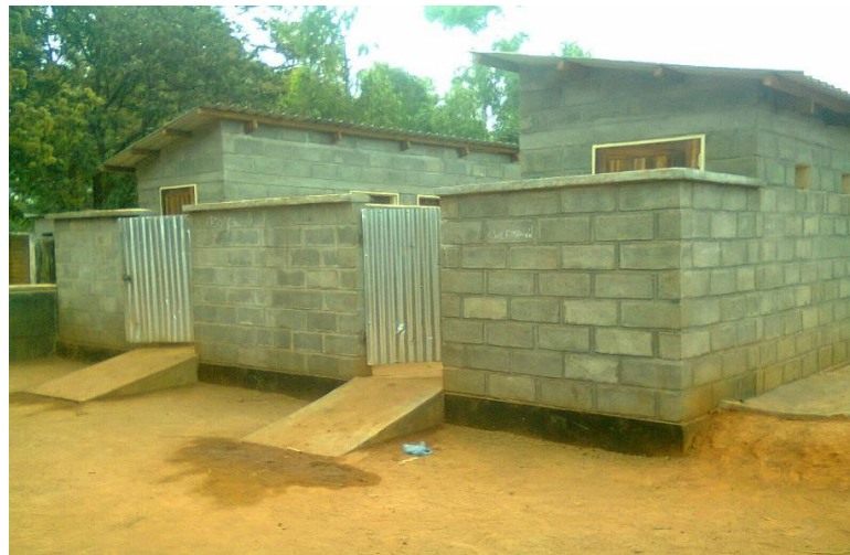
Figure 4: Quality latrines with access ramps for physically challenged learners
